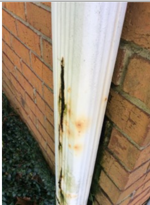
Damaged downspout
