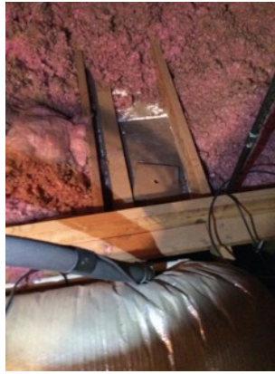
Missing insulation
