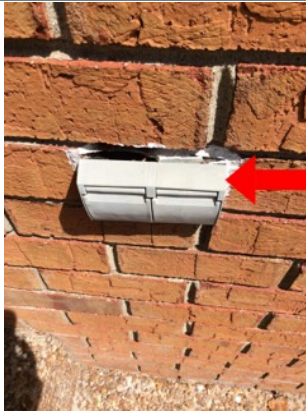
The rear exterior outlet is loose. Secure the outlet and cover to the electrical box.
