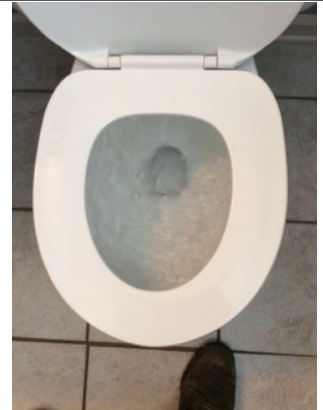
The toilet in the half bathroom is loose. Secure the toilet to the floor. The toilet also flushes slowly.
