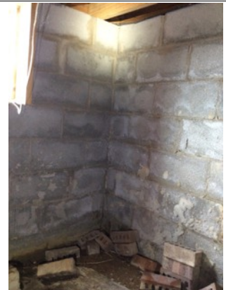
Moisture stains and effervescence was seen on some of the foundation walls.
