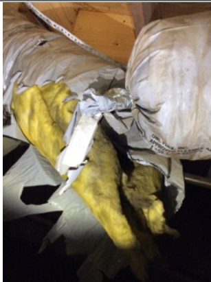
A disconnected HVAC duct was found in the crawlspace. Repair the duct.
