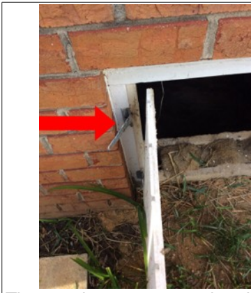
The crawlspace access door is damaged. Repair or replace the door.
