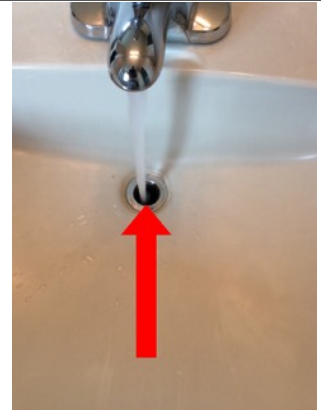
The stopper for the master bathroom sink is missing. Add a stopper to the sink.
