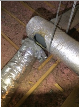
Disconnected duct
