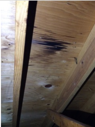
Moisture stains were seen on the roof sheathing.
