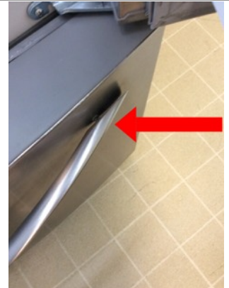
The freezer door handle is loose. Repair the handle.
