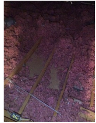
Missing insulation
