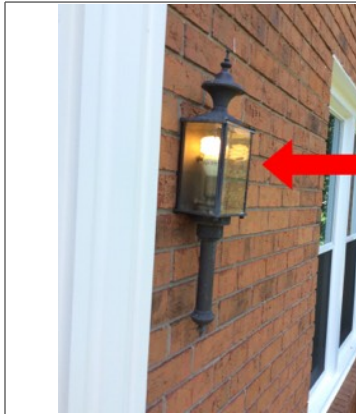
The exterior lights by the front door are loose. Secure the lights to the electrical box.
