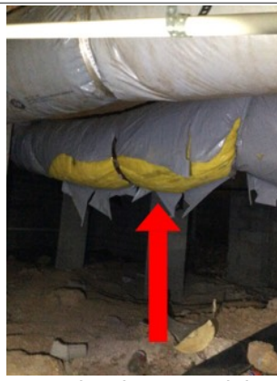
The vapor barrier around the crawlspace HVAC ducts is damaged. Repair the ducts.
