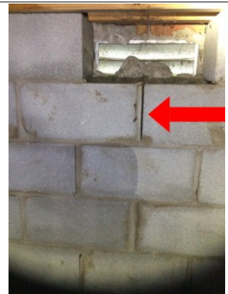
Small cracks were seen along the front wall of the crawlspace. Seal/repair the affected areas.
