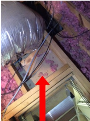
Insulation is missing in multiple areas in the attic. The insulation base varies from 2-6 inches deal. Recommend adding additional insulation to the attic.
