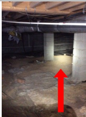
A vapor barrier is missing in parts of the crawlspace. Add a vapor barrier to the affected areas.
