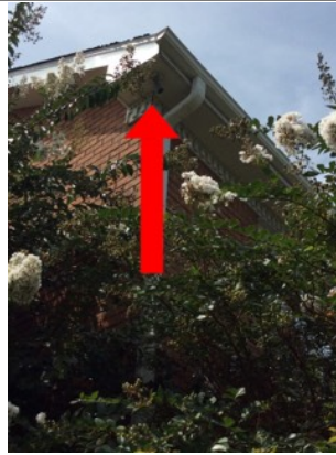
The exterior flood lights have no light bulbs. Add bulbs and test.
