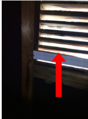
A screen is missing on the south side gable vent. Add a screen to the vent.
