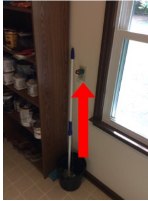
An outlet in the laundry room is loose. Secure the outlet to the electrical box.
