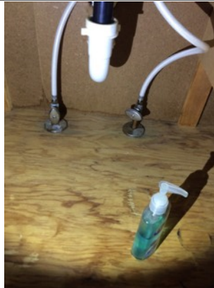
Moisture stains were seen on the base of the vanity in the half bathroom.
