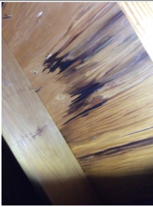
Staining on the roof sheathing.
