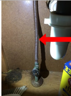
The water line under the master bathroom sink has rusted. Replace the line to help prevent future leaking.
