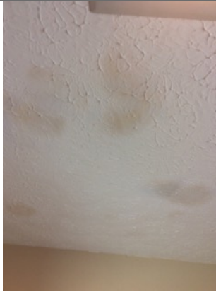
Moisture stains were seen on the ceiling of the bonus room.
