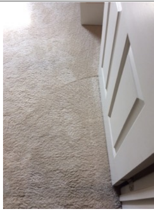
The west bedroom door is rubbing on the floor.
